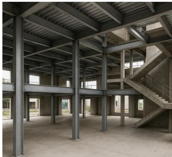
Typical Type IIB Construction
